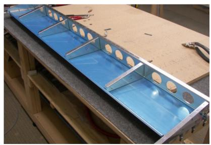
Conventional Spar and Rib Construction. Traditional spar at top, bottom skin is folded at rear to form a faux rear spar providing an attach point for ribs trailing edge.
